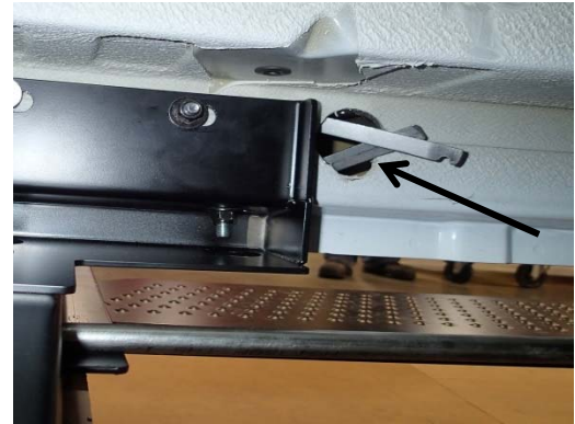
Tighten all hardware. Take the excess bracket material and bend it so you are able to get all the metal into the 1.5" hole.
