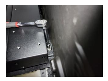
Tighten floor bracket hardware.
