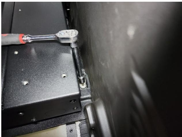
Tighten floor bracket hardware. Attach side top trim brackets with 1/4" x 3/4" Hex bolts and star washers.
