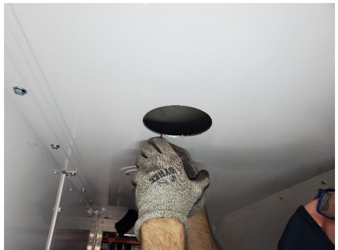
Deburr the hole in the ceiling to eliminate rough edges.
