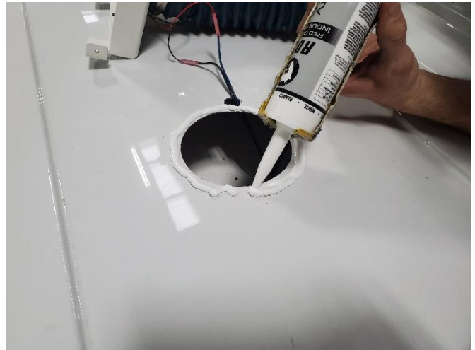
Caulk around holes on vehicle roof.
