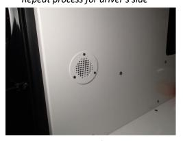
Attach round vent to front wall using three (3) #10 x 1/2" flat head screws and Keps nuts.
