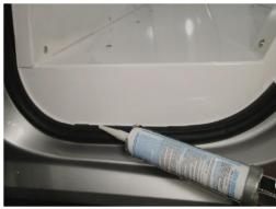
Silicone the lower seams to create proper water drainage.
