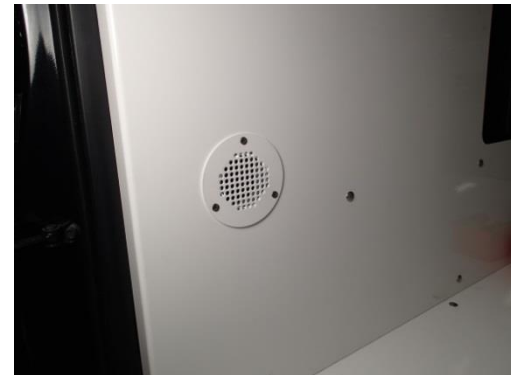
Attach round vent to front wall using three (3) #10 x 1/2" flat head screws and Keps nuts.
