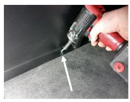
Place bottom of partition against bottom of seat and attach to floor with 1/4" x 1" lag bolts.
