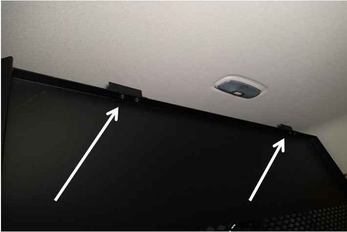
Attach the upper partition brackets to the upper partition base using four (4) 1/4 x 3/4" carriage bolts and serrated nuts.
