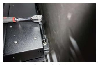
Tighten floor bracket hardware.
