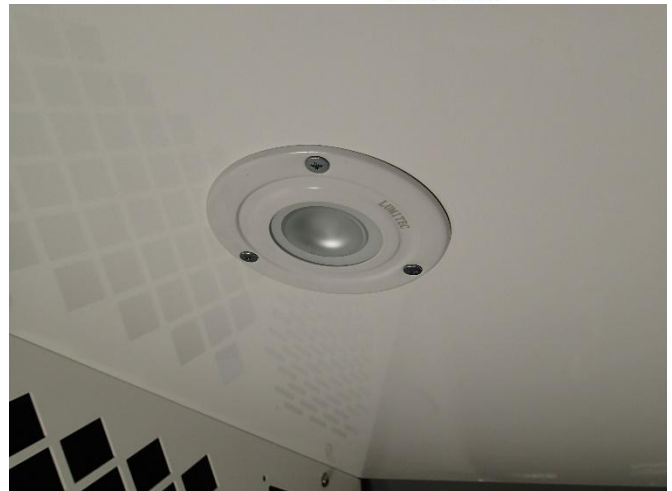
Install LED dome light as per instructions and hardware included with the dome light kit.
