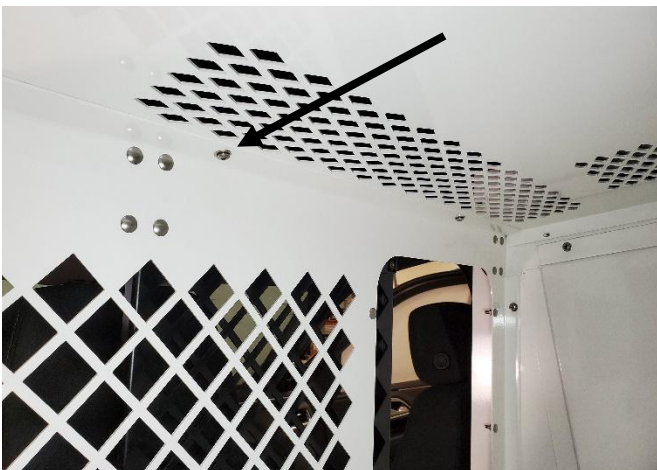
Attach ceiling to front bulkhead using 1/4" x 3/4" Phillips head bolts and flat washers.
