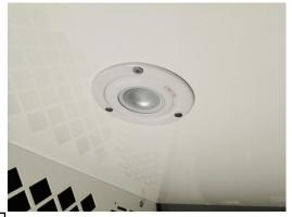
Install dome light in ceiling with #10 x ¾" flat head sheet metals screws included with dome light kit.
