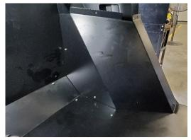
Place lower corner trim panel in and attach using 1/4" x 3/4" Phillips head bolts and washers.
