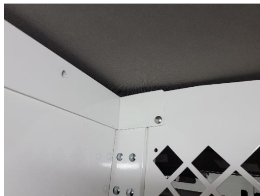
Attach filler to front bulkhead using 1/4" x 3/4" carriage bolt and nut.
