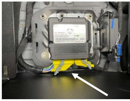
**Be careful not to damage OEM plugs and harnesses on transmission hump**
