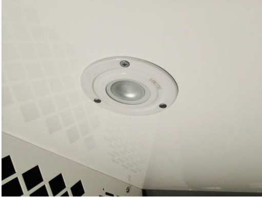
Install dome light in ceiling with #10 x 3/4" flat head sheet metals screws included with dome light kit.
