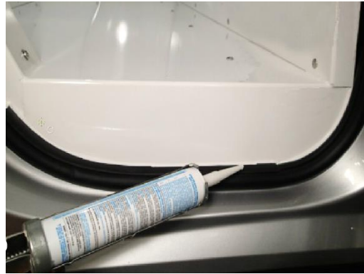
Silicone caulk all lower seams to ensure a watertight seal.
