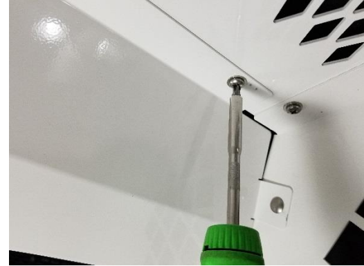
Place the upper trim panels in the kit and attach using 1/4" x 3/4" Phillips head bolts and washers.
