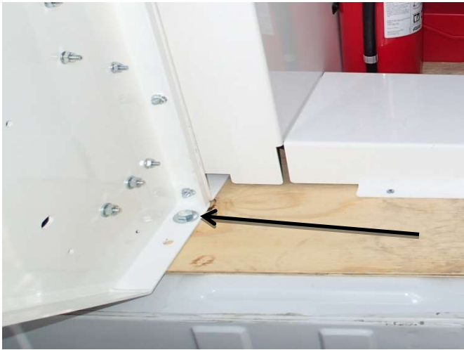
When bolting the front bulk head through the floor use the inner hole as shown.
