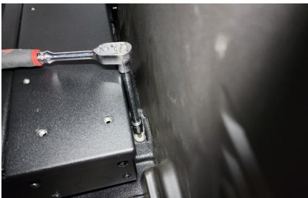
Tighten floor bracket hardware.
