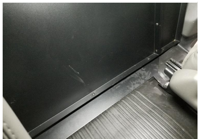
P-MFK-4 Only Attach to the lower mounting bracket using 1/4" x 3/4" carriage bolts and serrated nuts.
