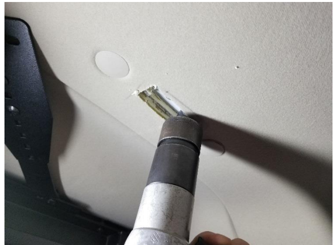
Install 1/4"-20 Rivnuts using Rivnut gun or other Rivnut tool.
