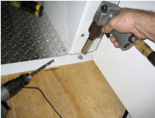
Remove the temporary # 10 screws and drill a 3/8" hole in the corners of the kit for through bolts.
