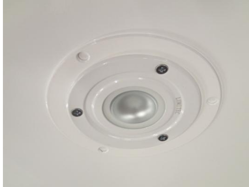
Wire and mount dome lights in ceiling cutouts
