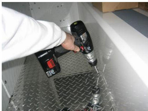
Using a screw gun, install #10 x 1.25" Phillips pan head screws into the floor.
