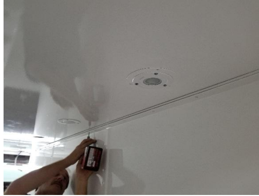
Repeat process for ceiling.
