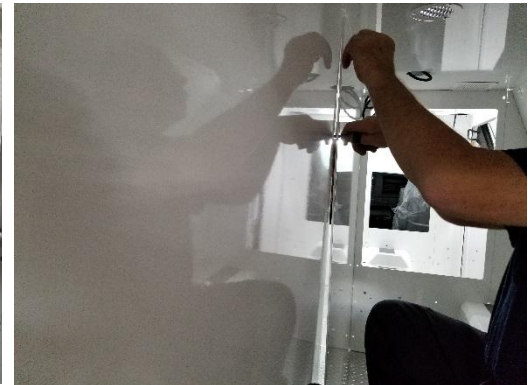
Attach divider sections together with 1/4" x 5/8" stainless socket button head bolts and washers.
