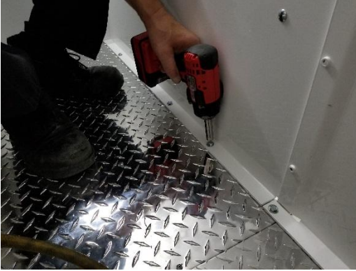
Attach divider to floor with 1/4" x 1.25" #14 lag bolts.
