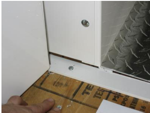
Drill and temporarily attach the rear lower corner of the door frame with a #10 Phillips sheet metal screw.
