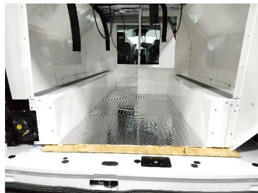
Slide main floor assembly into van and line up to the forward floor. Floor should be sitting on top of lip on benches.
