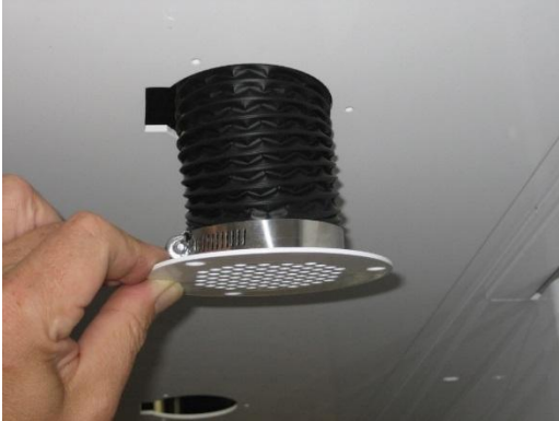
Attach vents to the vent covers with supplied hose clamps.
