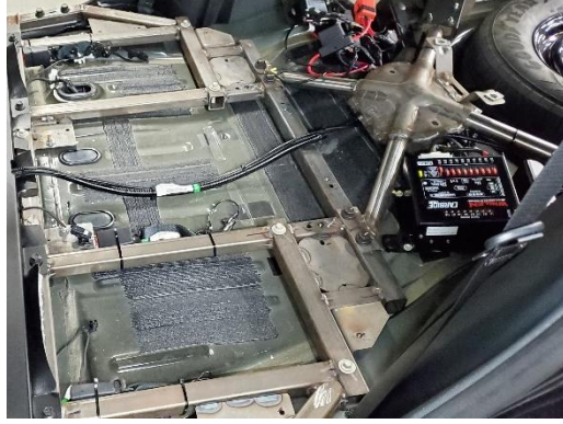
Remove back seats and set aside. Hardware will be reused.
